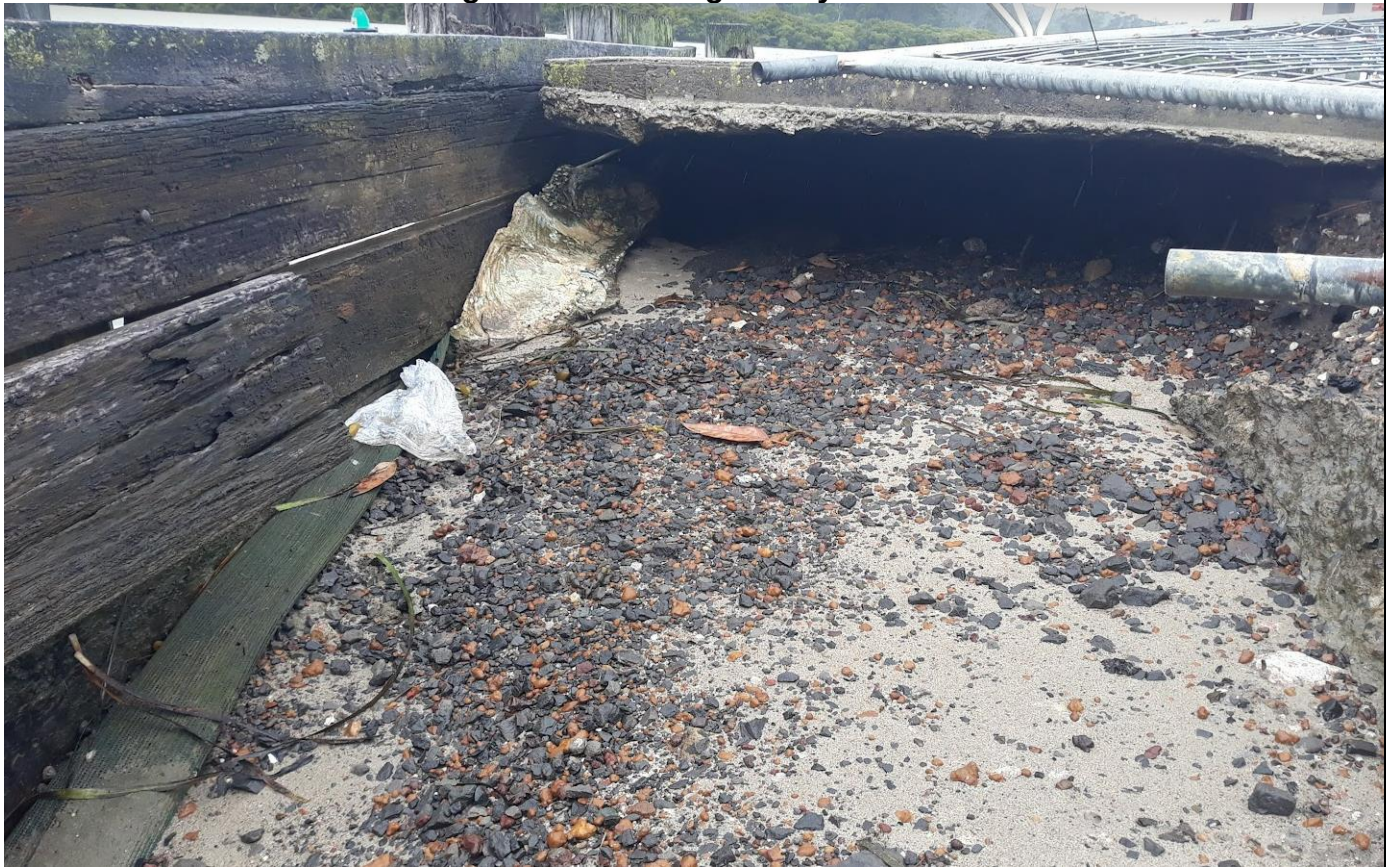
Photo 4: Extent of undermining of fish cleaning facility slab
