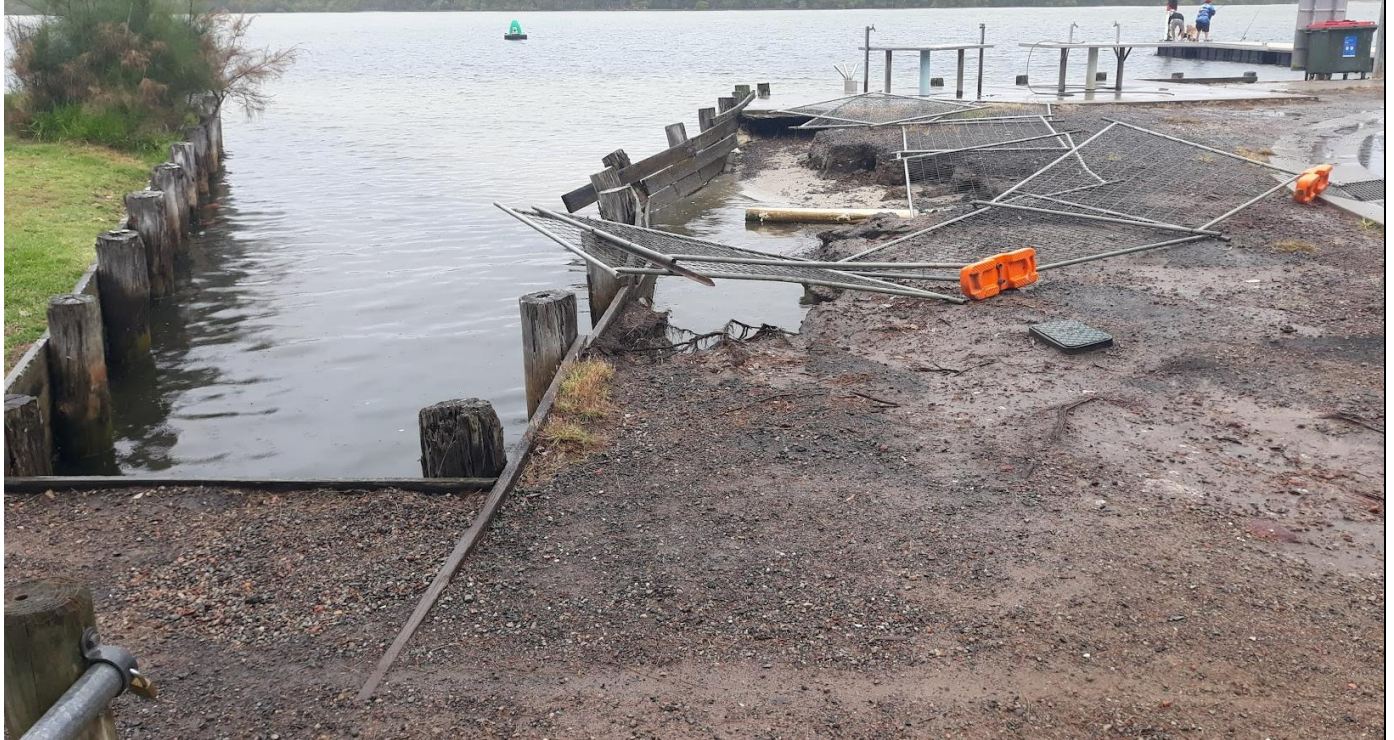
Photo 2: Damaged retaining wall to be replaced and gravel pavement. Also showing Swamp Oak regrowth (left-hand side of the photo) that would not be affected.
