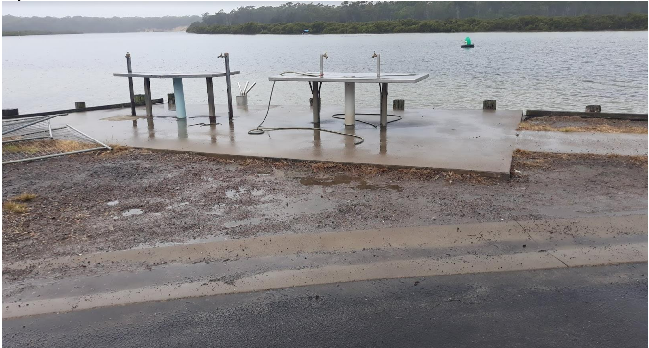
Photo 4: Extent of undermining of fish cleaning facility slab
