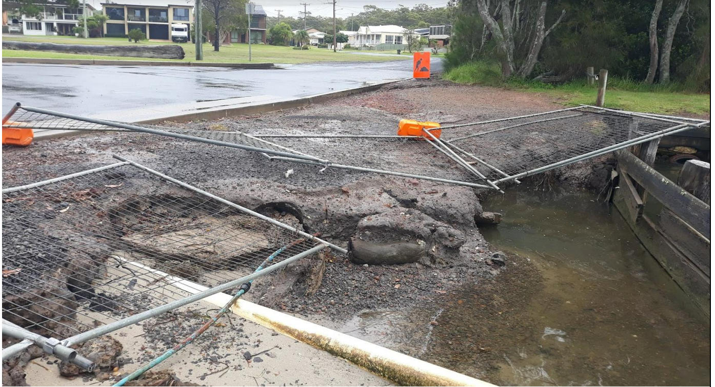
Photo 2: Damaged retaining wall to be replaced and gravel pavement. Also showing Swamp Oak regrowth (left-hand side of the photo) that would not be affected.
